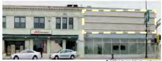
Existing large blank wall area
