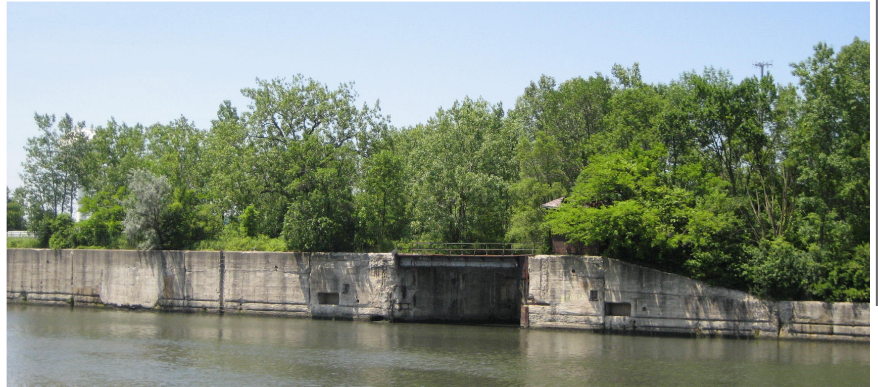
VIEW OF THE NORTH LOCK WALL FROM FAY'S POINT
