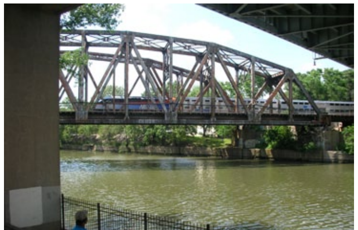
Blue Island's bridges and the Rock Island Metra service can help integrate the outlying California Gardens neighborhood south of 139th Street with Uptown and the Cal-Sag Trail. Photo: Charles Crump/URS.
